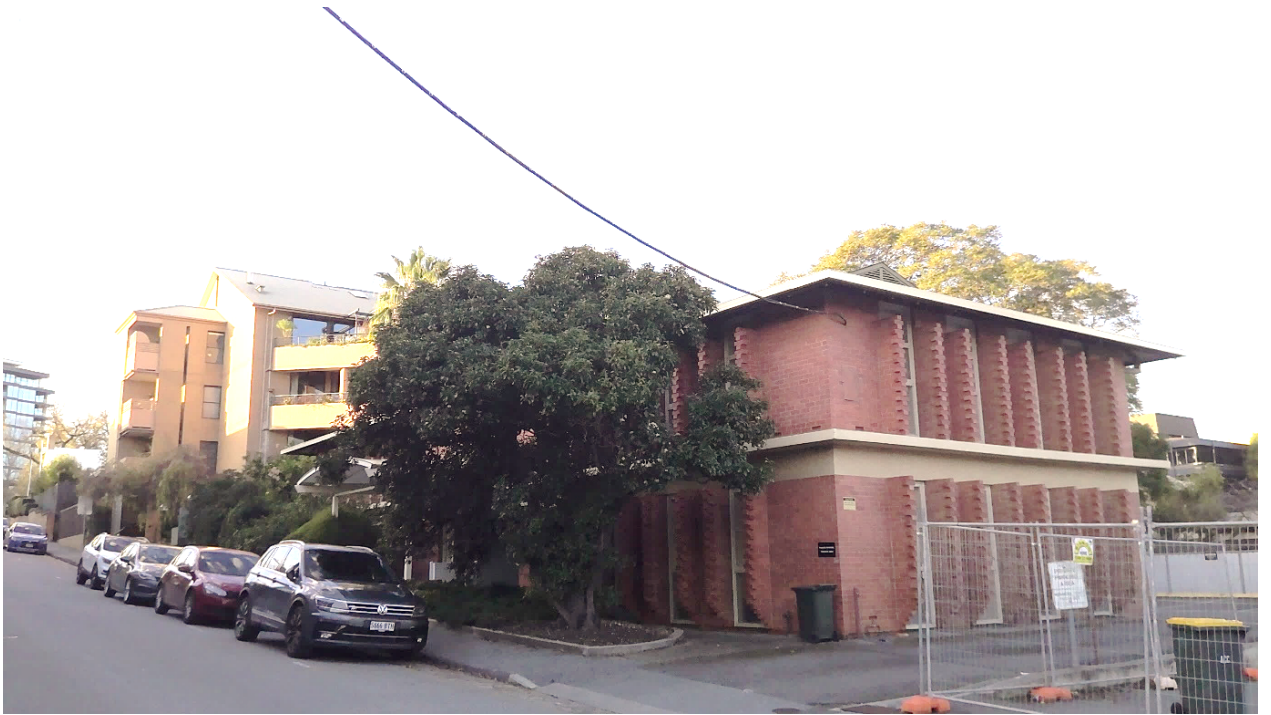
Figure 3.6 – Eastern side of Bagot Street looking north
