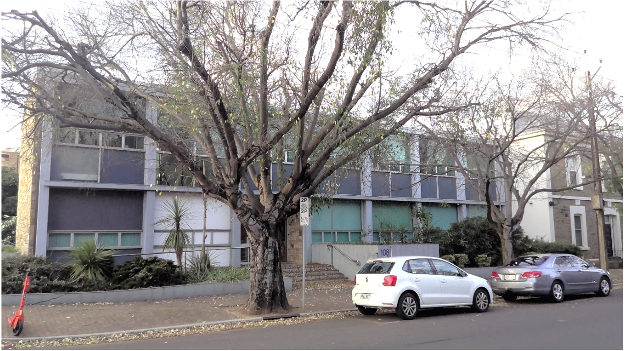
Figure 3.1 - Subject site viewed from Kermode Street
